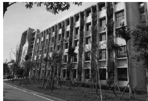
FIGURE 5 South side outer wall vertical greening
