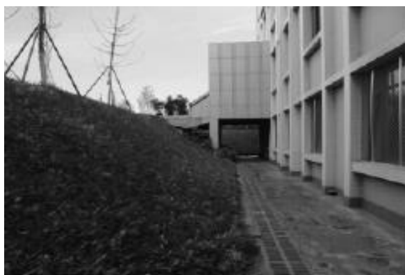
FIGURE 3 Slope greening that meet basement lighting requirement
