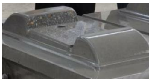
FIGURE 1 Grinded bearing rail platform
