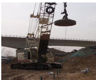
FIGURE 1 The site of dynamic compaction construction
